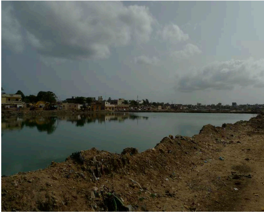
Figure 7.4: Retention pool Nietty Mbar (photo: author)
