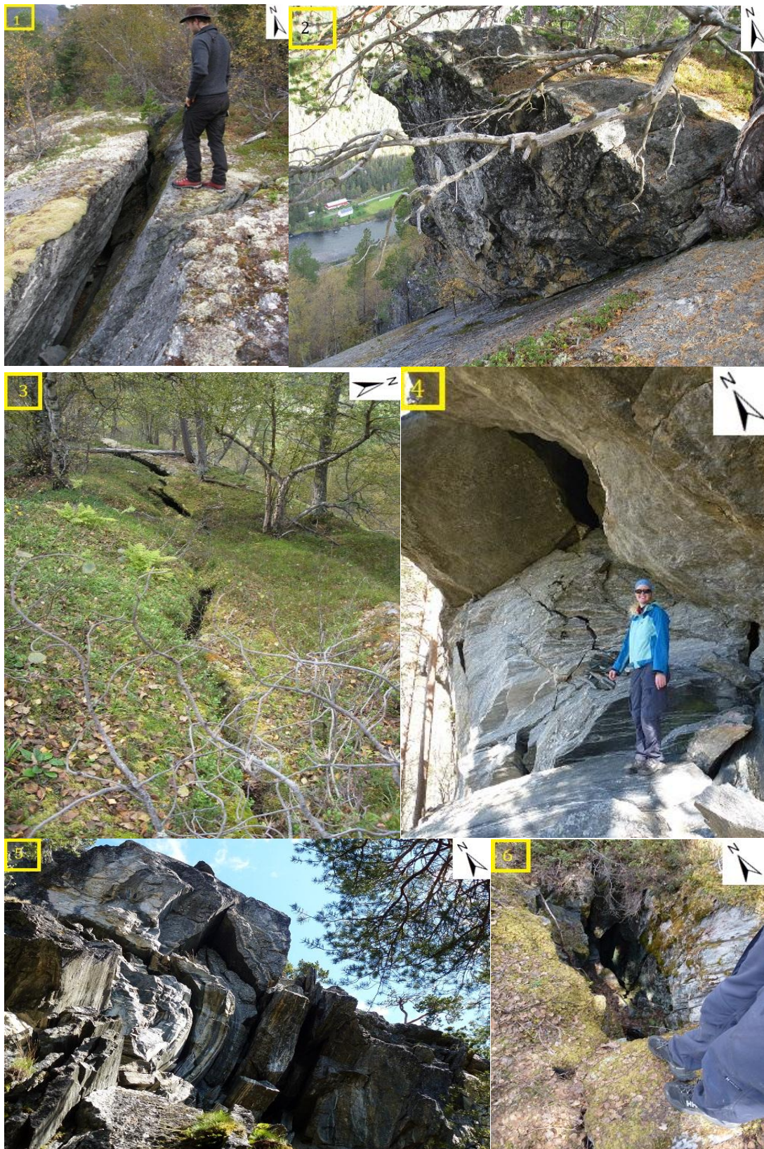
Figure 33 Picture 1 and 2 and is from the historical rockslide, picture 3 is in the middle of the historical and the unstable part, and figure 4,5 and 6 is taken from the unstable part at Ivasnasen. They all shows sign of activity with huge cracks and deformations. Pictures taken by the author.
