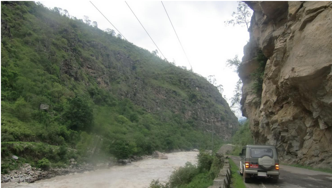
Figure 3.4 Location of final dam axis ( Google earth 3/2012)
