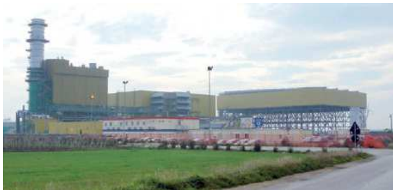
Figure 7.4 San Severo combined cycle plant (Ansaldo Energia)
