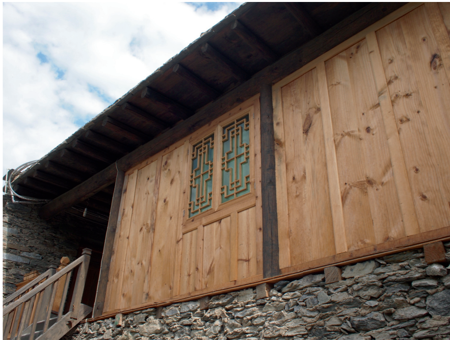
Figure 7. 4 The Former Storage Room Converting into a Guest Room
