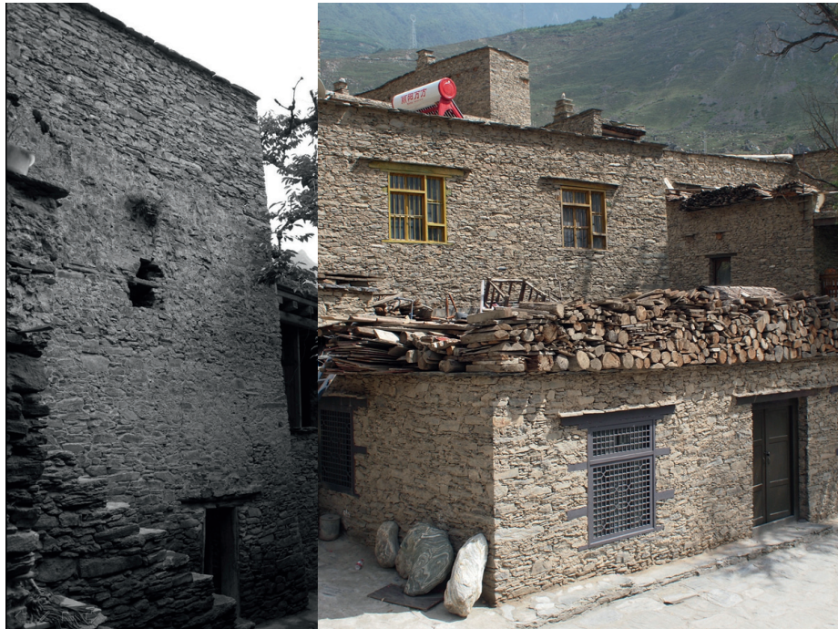
Figure 6. 9 The Enlarged Windows after the Self-restoration
