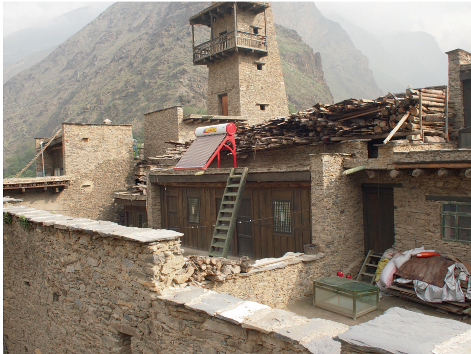
Figure 6. 10 The Former Storage Room Converted into the Guest Room
