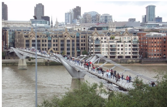
Figure 3.11: Millennium bridge in London experienced severe excitations during opening day in 2000.
