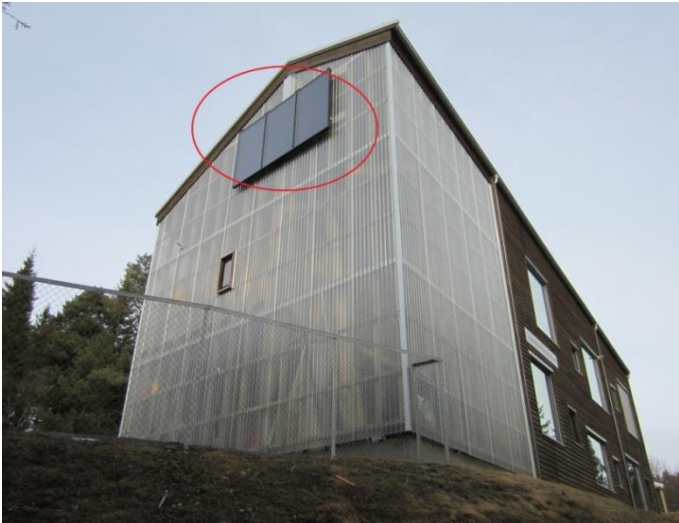
Figure 40 – Solar collector (red circle) placed on south-west facade
