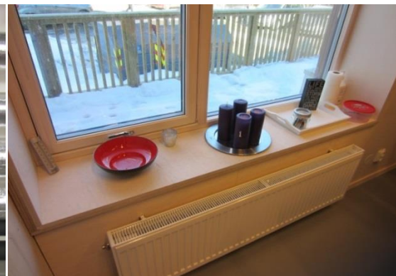
Figure 43 – Placing of radiators
