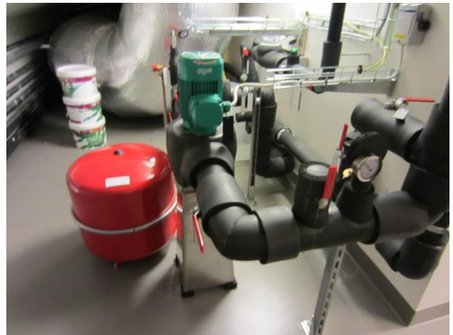
Figure 34 – Connection to bore holes
