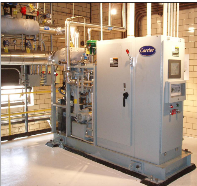
Figure 2. Euler Turbine package in parallel with a PRV station.
