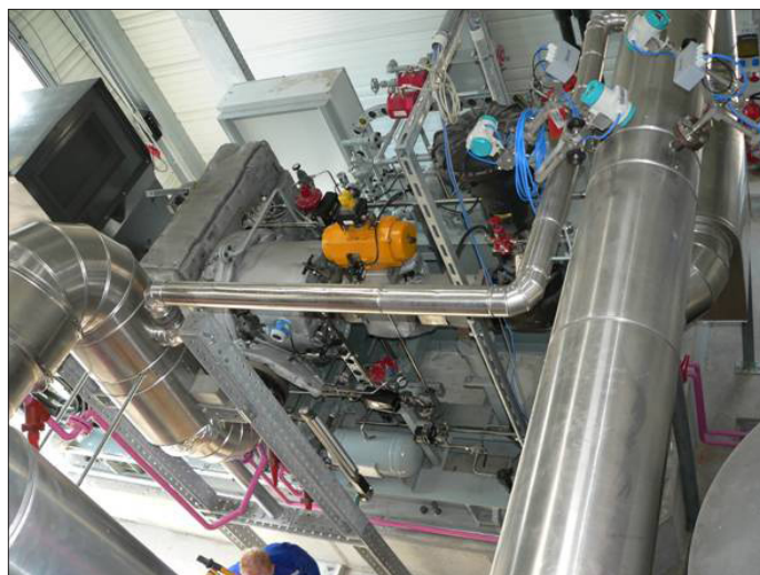
Figure 5. Model (top) and Installation (bottom) of the Euler Turbine skid for Kalina cycle geothermal power plant.
