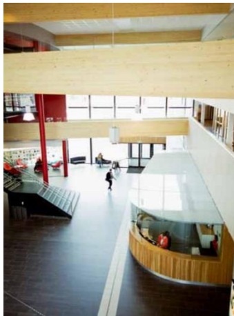
Figur 13: Terningen arena, brannimpregnert furu (AS, 2014)
