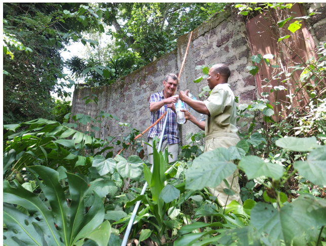
Figure 4.6: Filling the hose with water just below the hotel wall.
