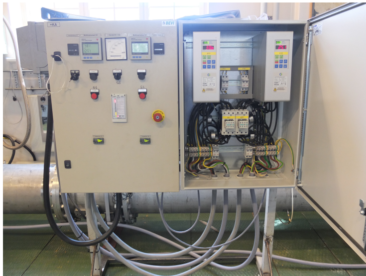
Figure 3.9: Cabinets for frequency controller and soft-start system. (Gjevik, 2014)
