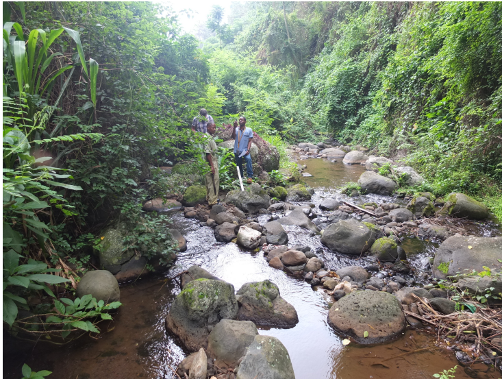
Figure 4.4: Intake and small dam from upstream.
