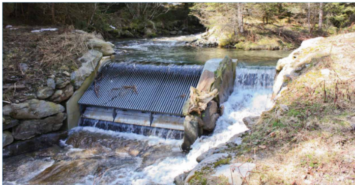
Figure 3.7: Coanda intake, 400 L/s. (Dahl, 2010b)
