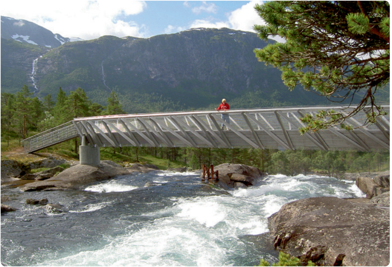
First walkwaybridge in LDX 2101® crossing Likholefossen at Gaularfjell in Norway.
