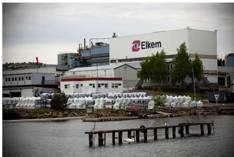
Figure 13: ELKEM Carbon Fiskaa plant
