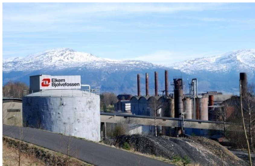
Figure 10: Elkem Bjølvfossen plant
