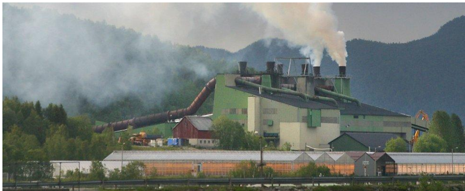
Figure 9: Elkem Salten plant
