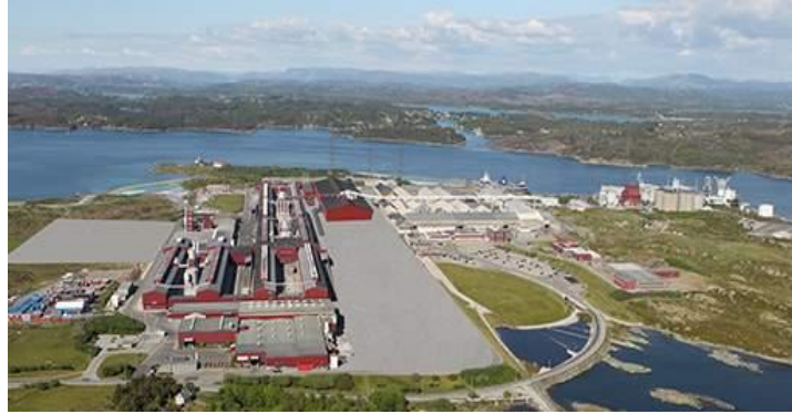
Figure 25: NORSK HYDRO Karmøy plant
