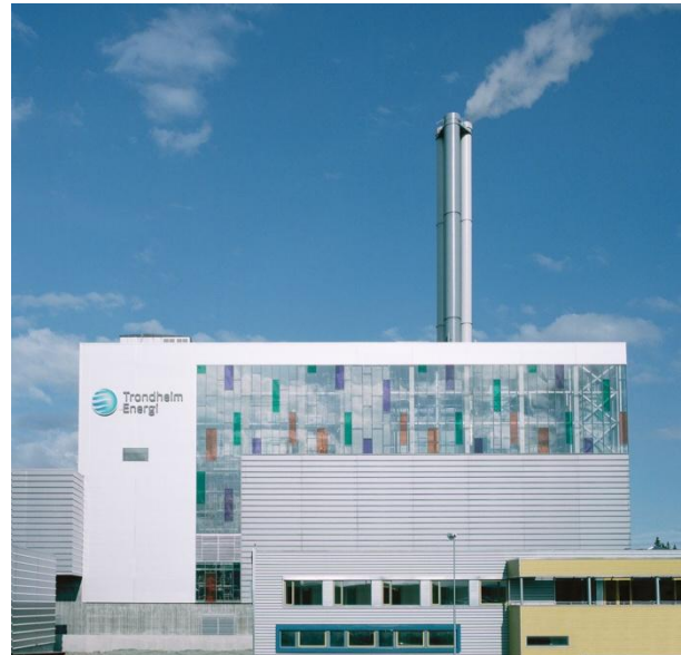
Figure 5: “HEIMDAL VARMESENTRAL” plant
