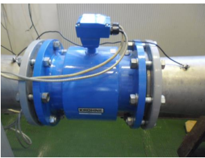
Figure 8: Installed electromagnetic flow rate meter.
