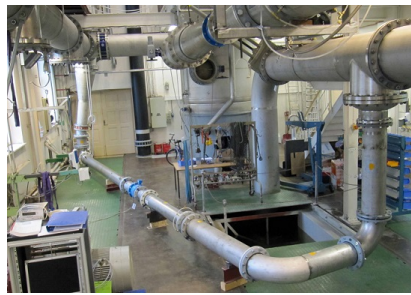
Figure 5.1.2: Rebuilding the piping system for calibration of flow meter
