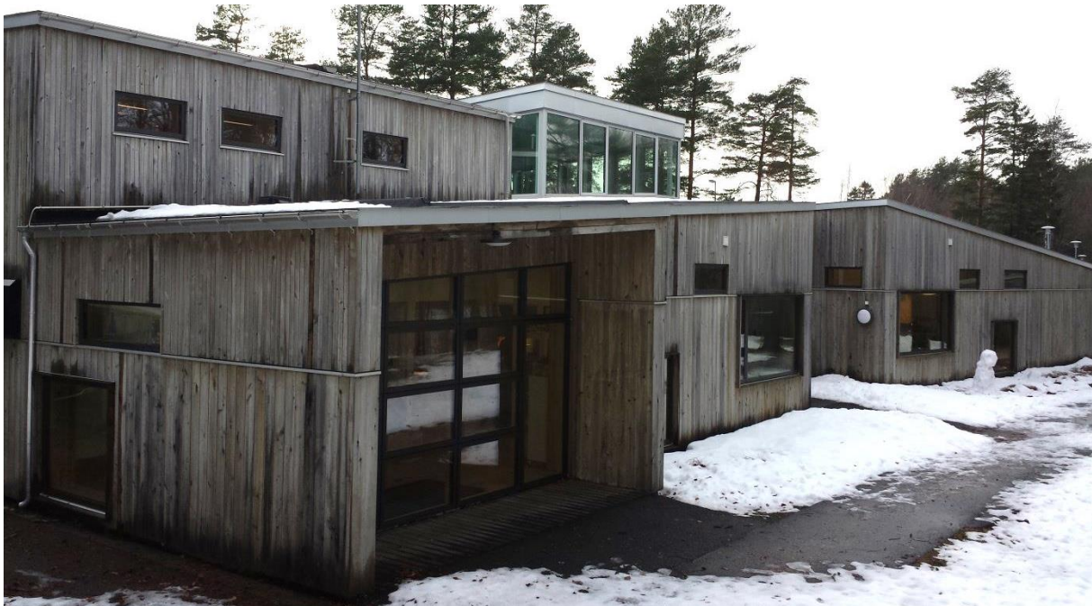
Figure 5.1: Picture showing the north façade of Solstad kindergarten.
