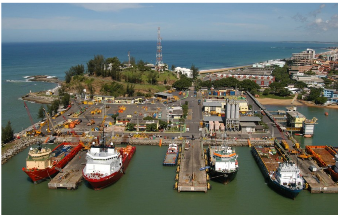
Figure 2-5: Imbetiba port at Macaé (Petrobras, 2013)
