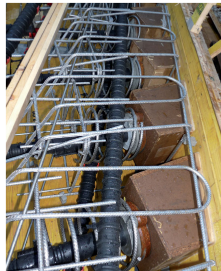
Figur 10.4: Spaltstrekkarmering for Egg-Graben Brücke [3, Fig. 10].
