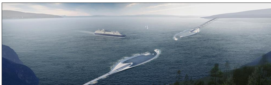
Figure 1-1: Illustration of proposal by Reinertsen AS and partners showing a fjord crossing by pontoon bridges and a submerged tunnel (Reinertsen AS, 2015)
