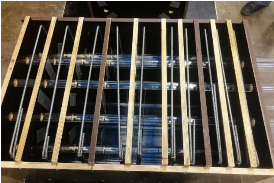
Fig. 44 Reinforcement bars inserted
