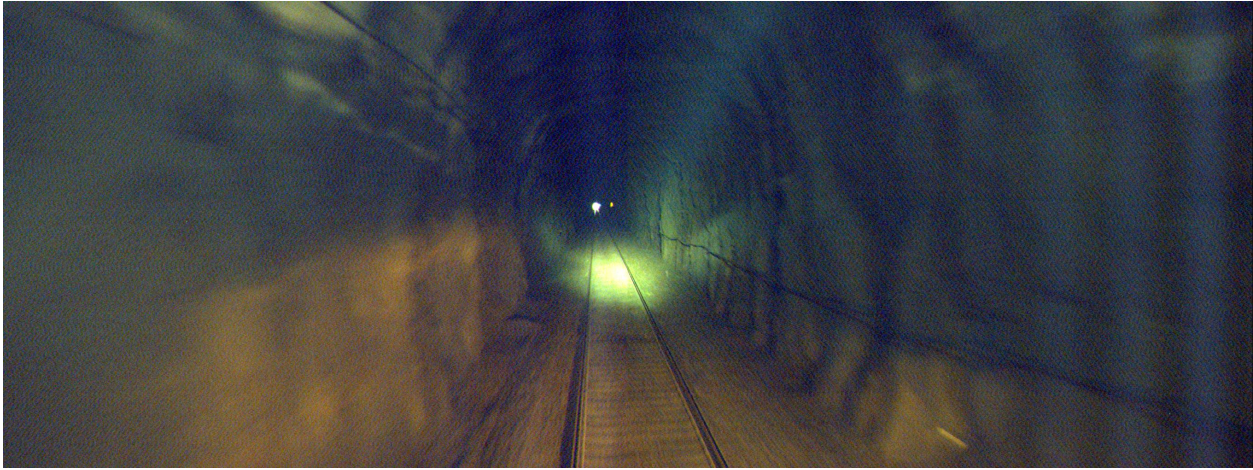
Figure A.8: Gylandtunnelen 451.209 km
