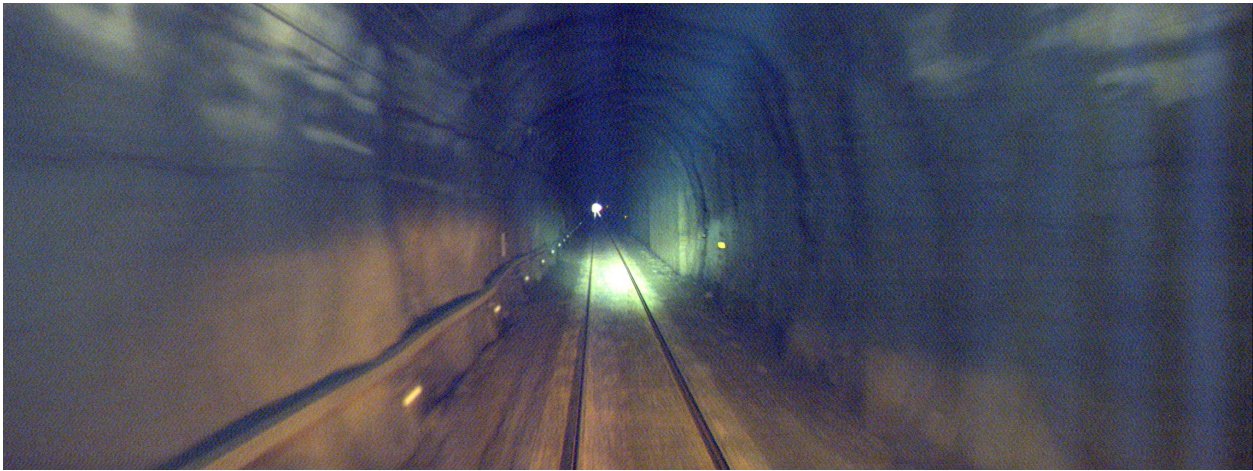
Figure A.9: Hægebostad at 427.116 km
