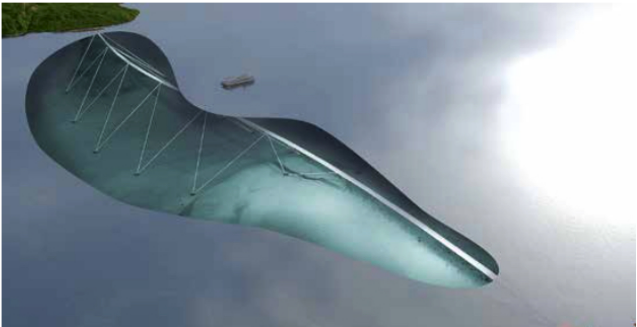
Figure 2.12: The submerged floating tunnel anchored to the seabed (SVV, 2012a)
