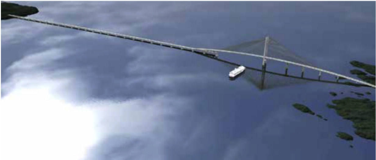
Figure 2.7: A suggestion of a floating bridge with end anchoring for Bjørnafjorden (SVV, 2012a)
