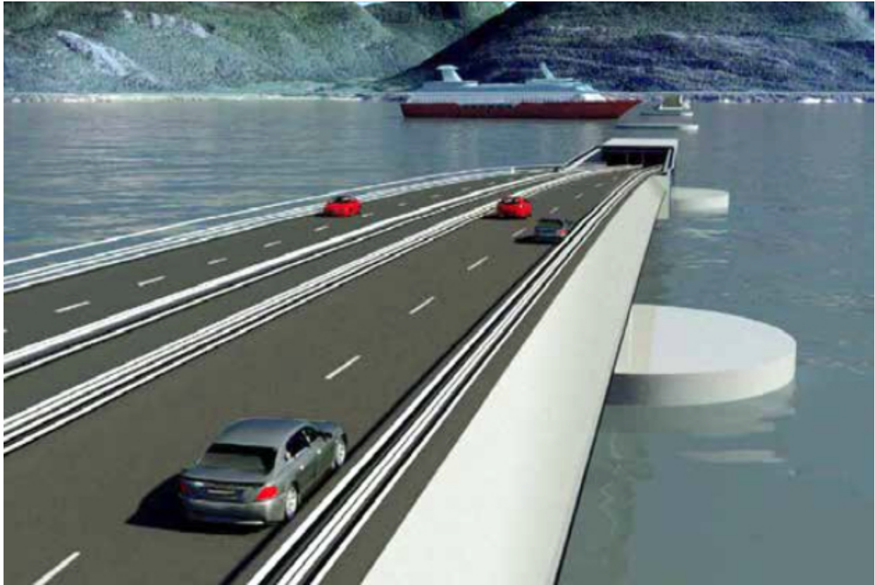
Figure 2.13: A combination of a submerged floating tunnel and a floating bridge ( SVV, 2012a )
