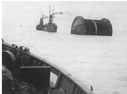
Figure 2-2 Laying Pluto in August 1944 after D-Day (beingbutmen.blogspot.no/)
