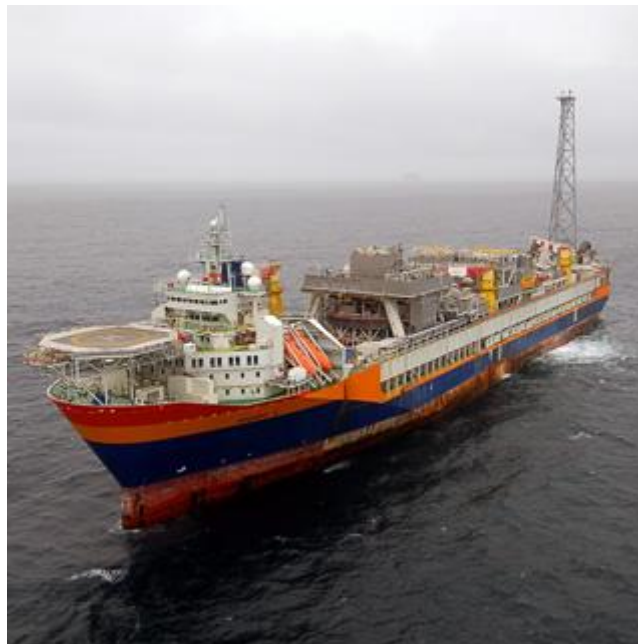
Figure 6-1 Åsgard A FPSO
