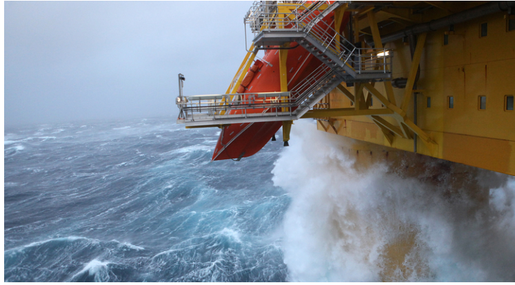
Figure 1.1: Free-fall lifeboat installed on an offshore installation, (PTIL, 2014)
