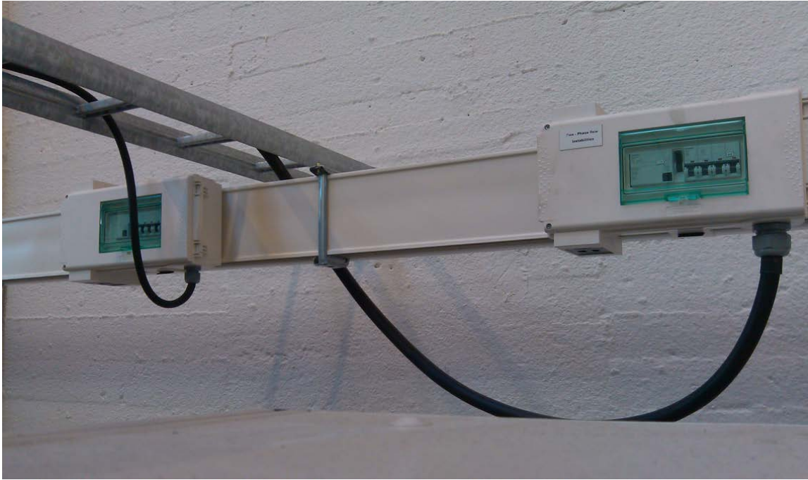
Figure 48: The contactors
