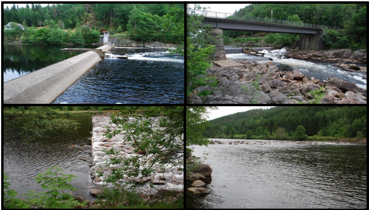
Figure 7. Weirs in Laudal bypass section (Mandalselva River). On the upper left corner Manflå Dam, upper right corner Kleveland concrete weir, both on the bottom are one of the 9 cobbles weirs view from two sides. Photos: Berit Köhler and Ana Adeva.
