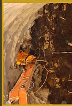
SCAVO DI TUNNEL TUNNEL EXCAVATION
