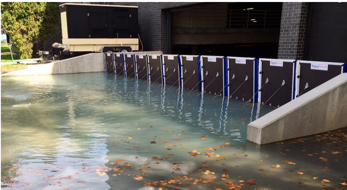
Picture 12: A flood barrier in use protecting an entrance to a warehouse
