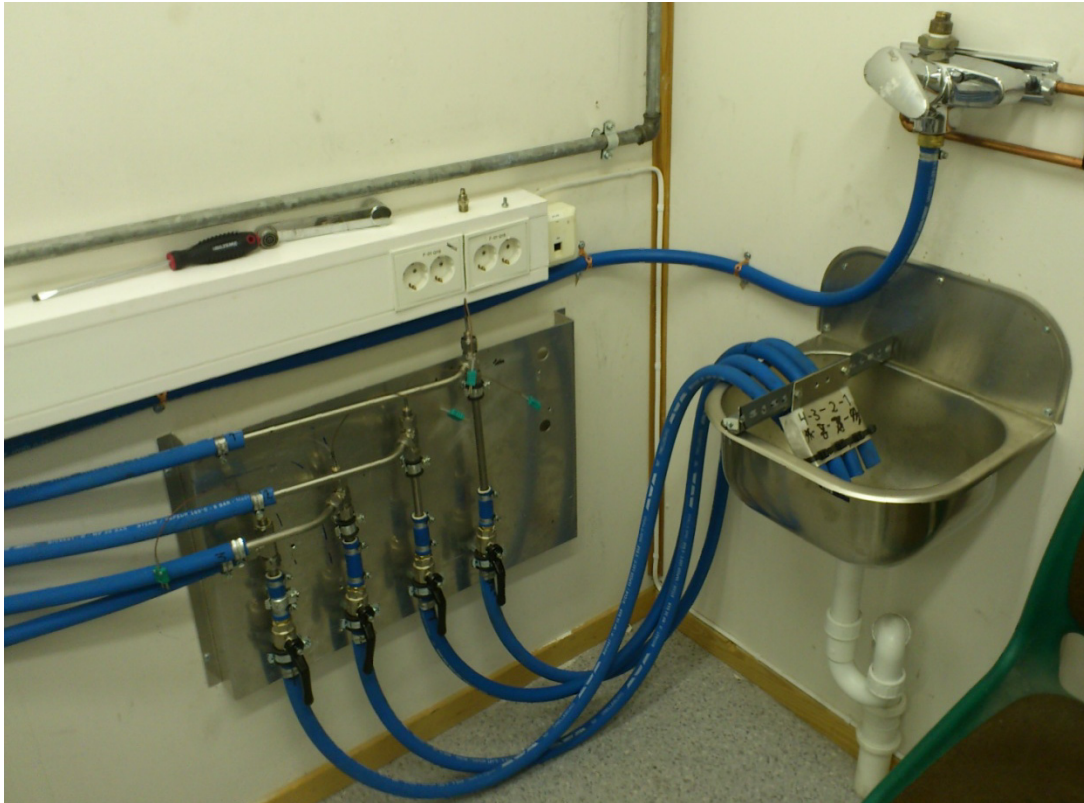
Figure II.35: Cooling system control panel, system inlet and system outlet.
