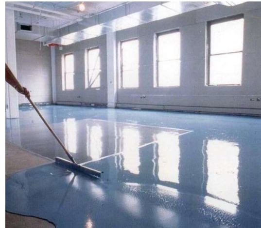
Figure 17 Epoxy floor (QLD, 2014)
