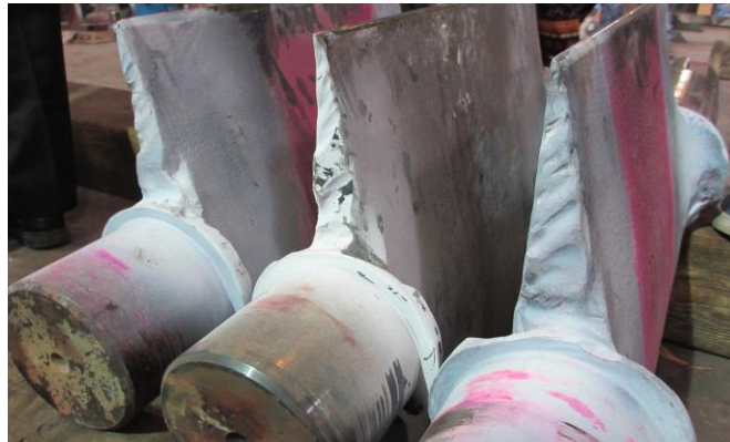
Figure 3 Eroded guide vanes from Kaligandaki power plant in Nepal (Writer's own photograph).
