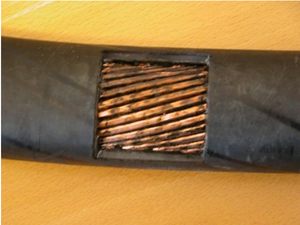
Figure 36: Large fault, 25cm 2 . [25]
