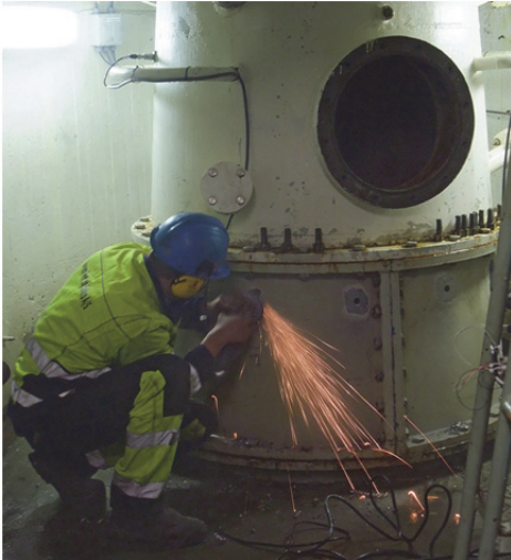
Figure 46 – Drilling holes and mounting pipe stubs on draft tube wall
