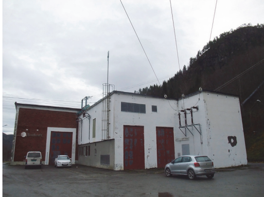
Figure 43 – Svorka Power plant
