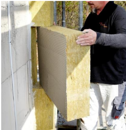
Figure 33. Application of Mineral Wool at the external wall.
