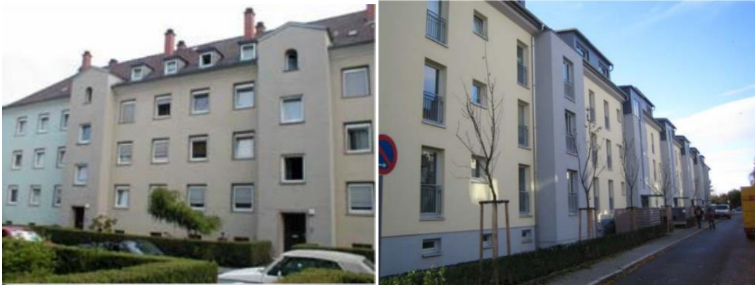
Figure 7. Blaue Heimat, Heidelberg - Germany. Before (left) and after (right) the renovation.
