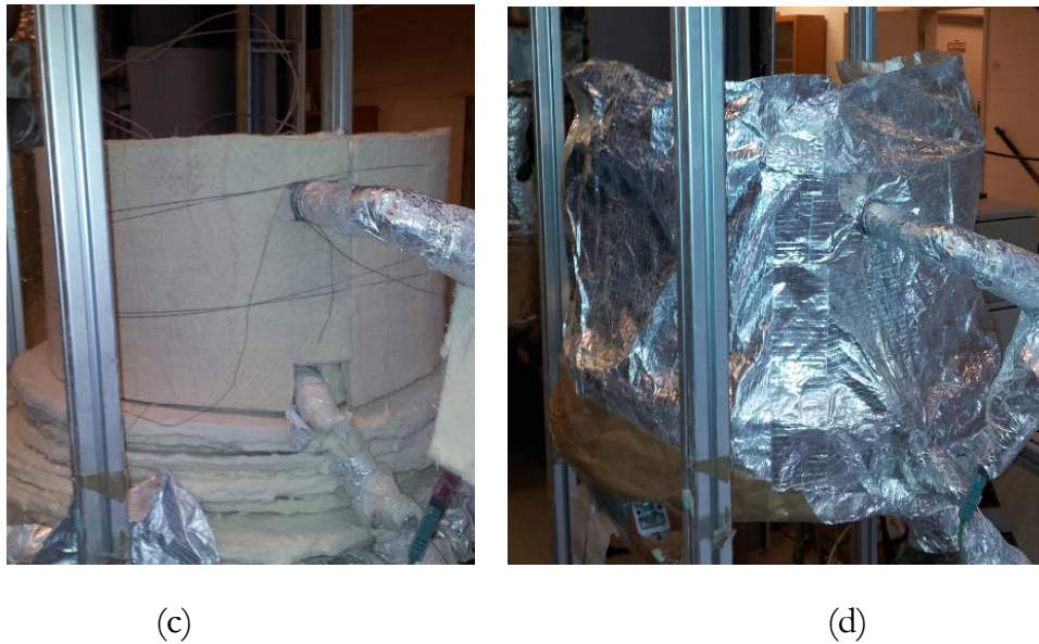
Figure 5.5: Application of insulation. (a-b) Horizontal view with and without upper lid. (c-d) Vertical view.
