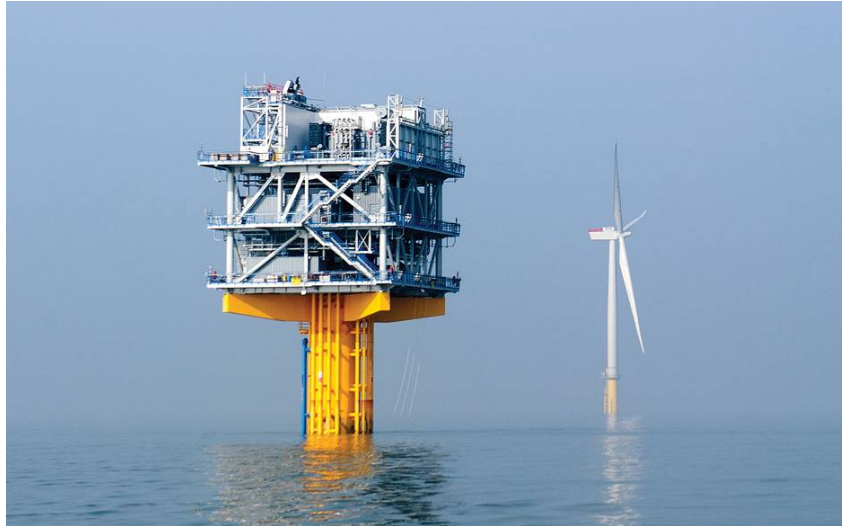
Figure 19: Offshore substation. The topside (grey) and the beginning of the foundation (yellow) can be seen. [41]
