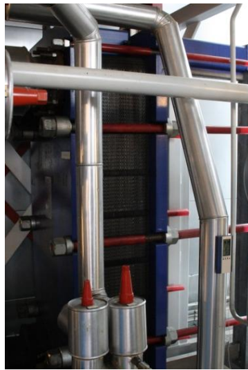
Figur 11. Platefordamper. Alfa Laval T20-BWFG.
