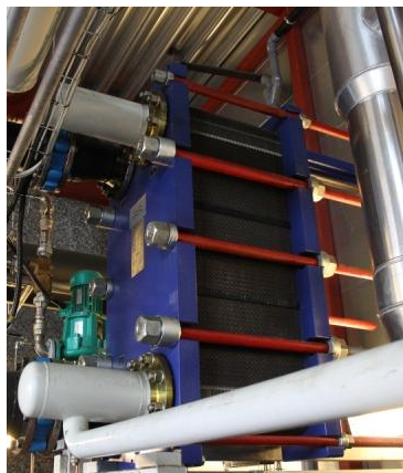
Figur 12. MT-kondensator. Alfa Laval MK15-BWFDR
