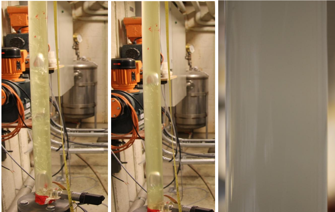
Figure 48: riser with water and bubble behavior due to instability
