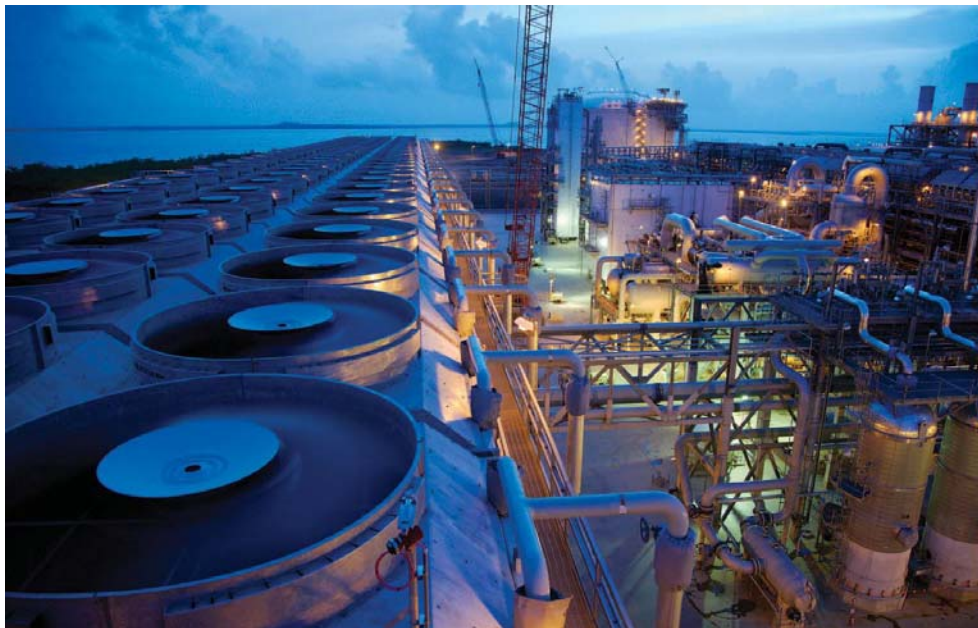
FIGURE 11 AIR COOLED PLANT (CONOCOPHILLIPS 2010)
