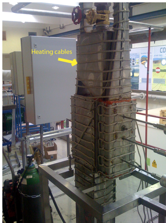
Figure 3.5: Filter tray heating cables.
