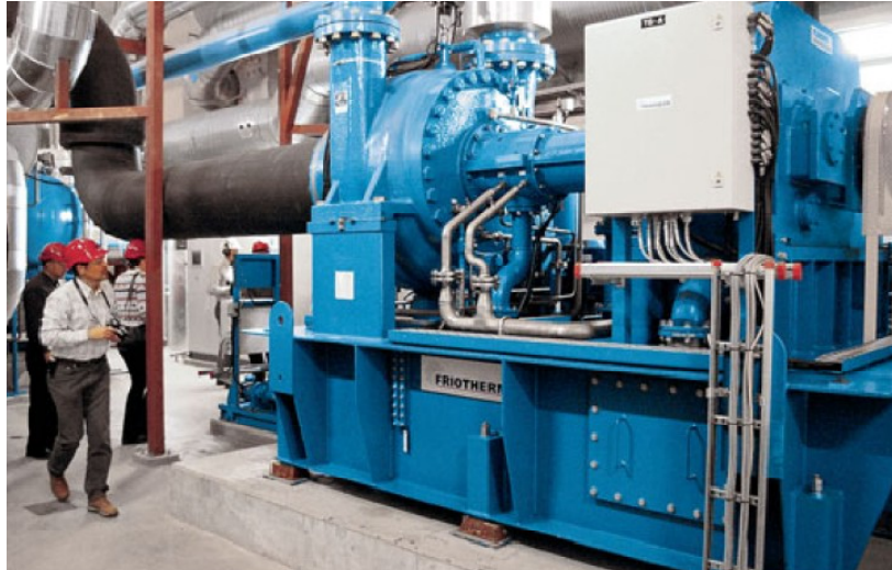
Figur 2-20 Turbokompressor Uniturbo 50 FY (Friothers AG, 2008)
