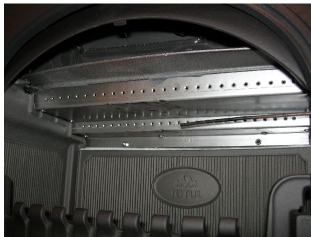
Figure 5.2: Secondary air system
