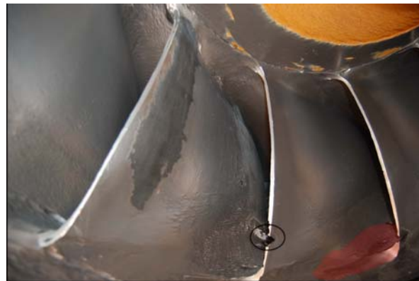
(b) Erosion at pressure side of blade
