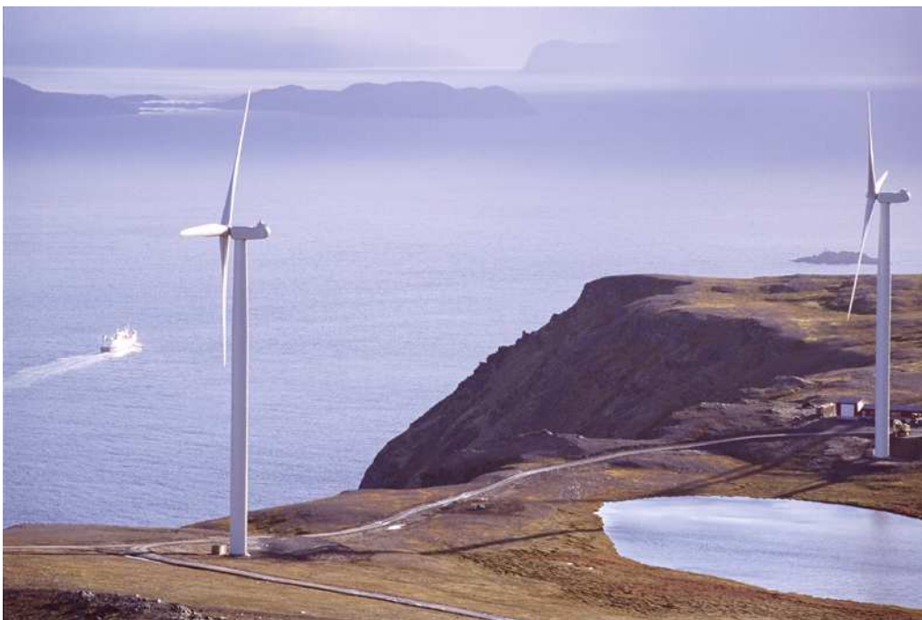
Figure 1.1: Photo from Havøygavlen in Finmark, Norway. The turbines are Nordex N80, with a rotor diameter of 80\text{ m} and installed capacity of 2.5\text{ MW} . Source: Nordex GmbH.
