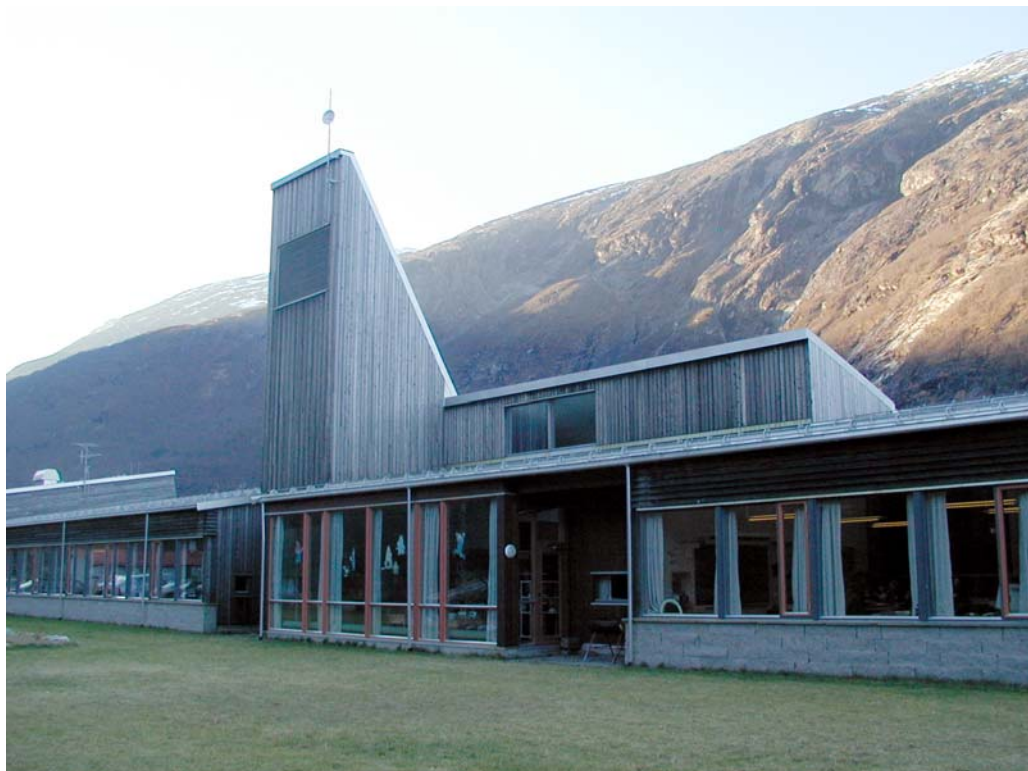
Figure 2. Tredal Primary School with its exhaust tower.
