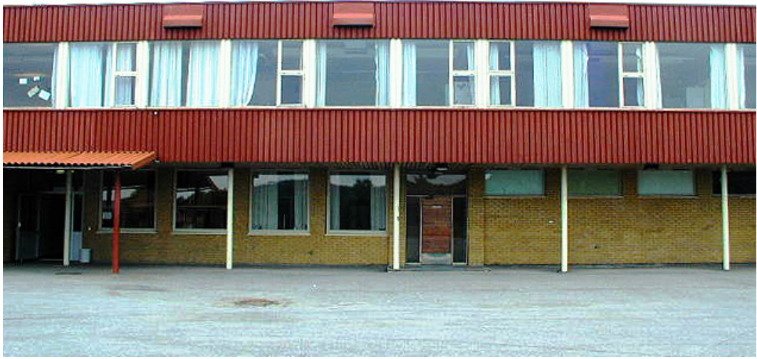
Figure 1. Separate air intake in the façade at ceiling level for each classroom.
