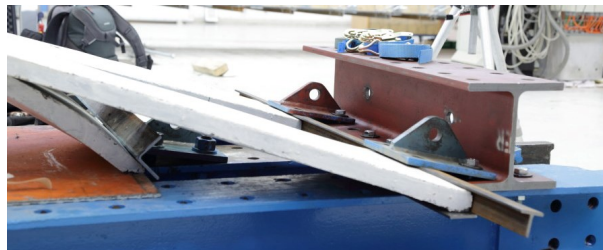
Figure 7.5: Outer ends fastened
