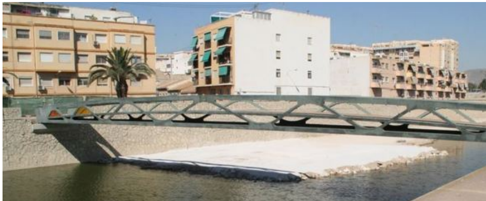
Figure 5.3: UHPFRC bridge over Ovejas ravine in Alicante
