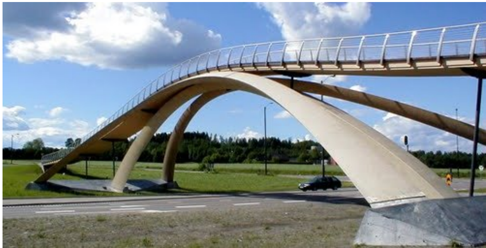
Figure 6.2: The da Vinci footbridge in Ås, designed by Aune Sand
