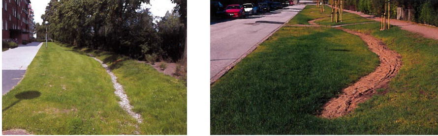
(a) Swale used as source control (Stahre 2006)
