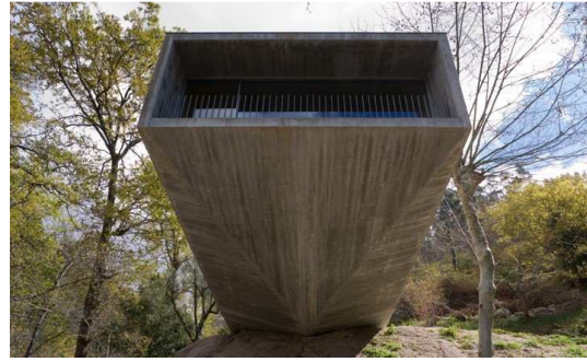
Figur 2.2-9: House in Geres, fasade mot vest [23]
