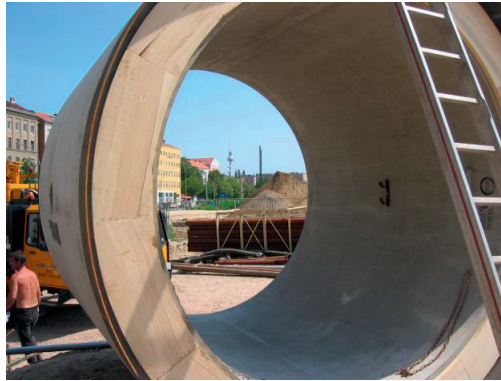
Figure 4 Reinforced concrete jacking pipe (inner diameter (ID) 2800 mm and outer diameter (OD) 3000 mm) (Photo:Tim E. E. Becker)
