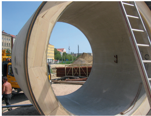
Figure 4 Reinforced concrete jacking pipe (inner diameter (ID) 2800 mm and outer diameter (OD) 3000 mm) (Photo: Tim E. E. Becker)
