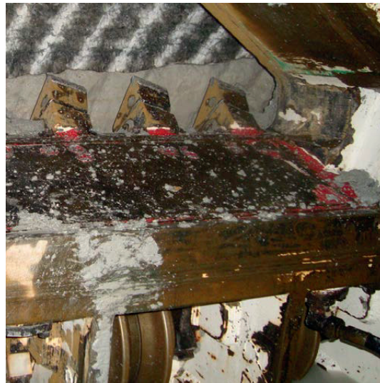
Figure 34. A soft ground face consisting of soft claystone (UCS < 2 MPa) and gypsum (UCS < 5 MPa).
