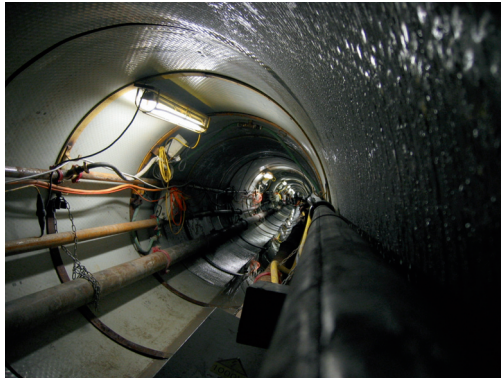
Figure 6 The Sammler Ost Tunnel (Photo: Tim E. E. Becker)
