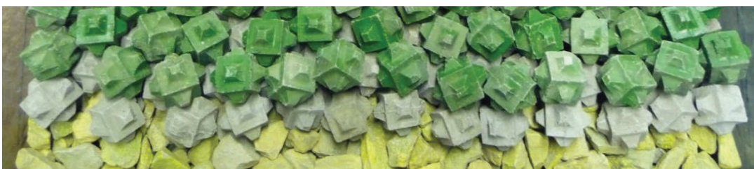
Figure 12. Detail of the placement of the first rows of concrete blocks
