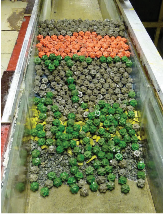
Figure 52. Breakwater after wave step four
