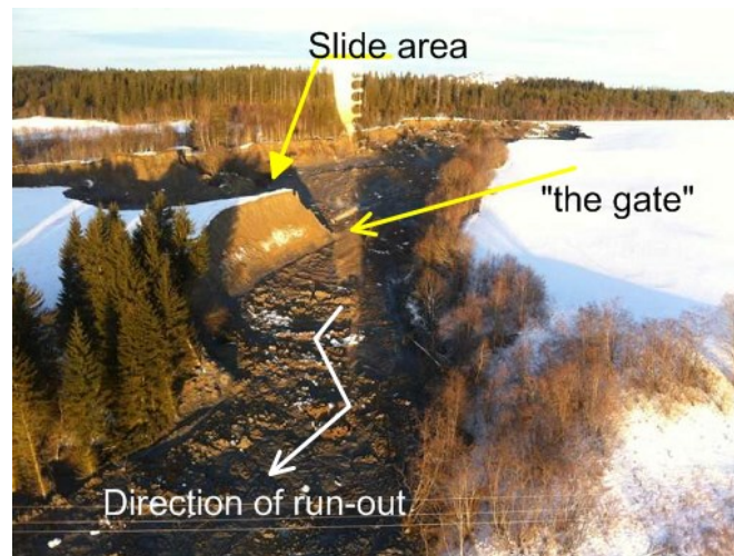
Figure 17 The Byneset flow slide (Source NVE, 2012). A closer view of the slide area and the gate.
