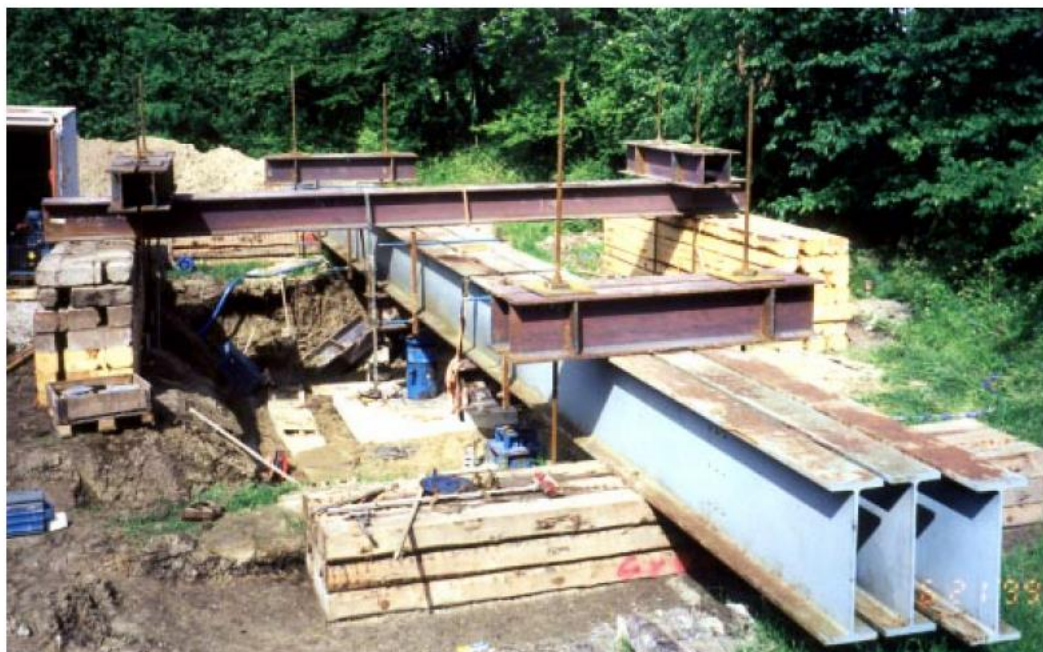
Figure 4.7 Reaction system being mounted at Tornhill footing load test site(Larsson 2001).
