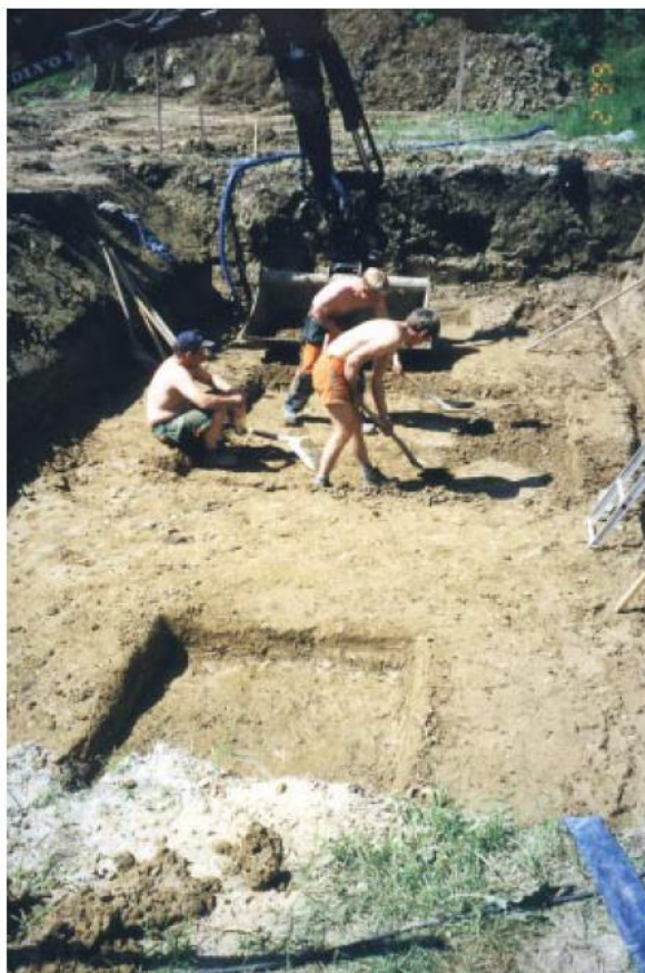
Figure 4.6 Excavation for the plates at Tornhill footing load test site(Larsson 2001).
